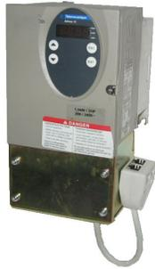
When the makeup air unit is direct gas fire (like the Spring Air Systems SAT unit) the supply drive can be located in the makeup air unit control panel or with the exhaust fan drive(s) in a separate enclosure. (SV Type)
